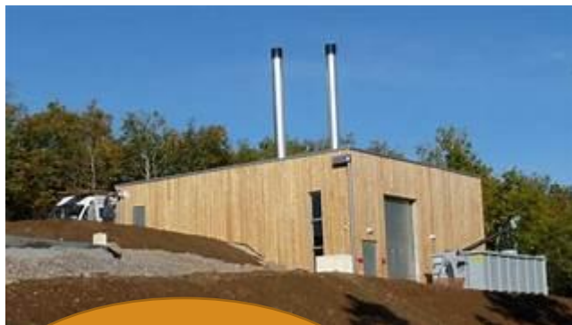
Chaufferie bois collective
